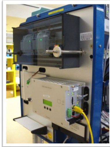
Figure 10: XSOS with power supplies (on top) and DCR-1 (below), and place for a VPN router (courtesy: EURATOM, Luxembourg).
