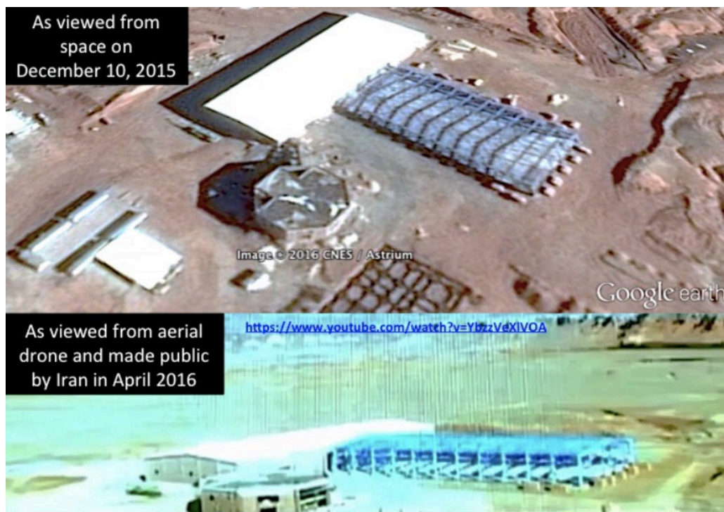
Figure 6: The Pasmangoor Nuclear Waste Stabilization and Storage Facility near Anarak, Iran. The white-roofed building is the concrete vault radiological waste storage building.
